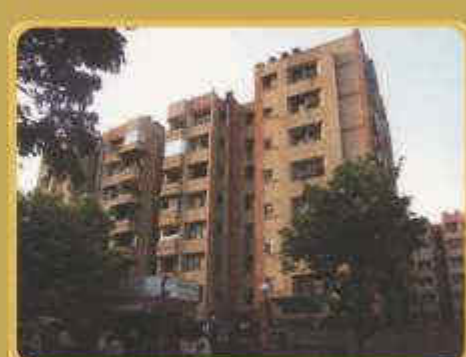
DSIDC Co-operative Apartments Plot 23, Sec - 9, Rohini Delhi Consisting 135 units
